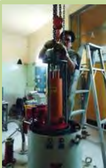
Klystron inspection and maintenance.
